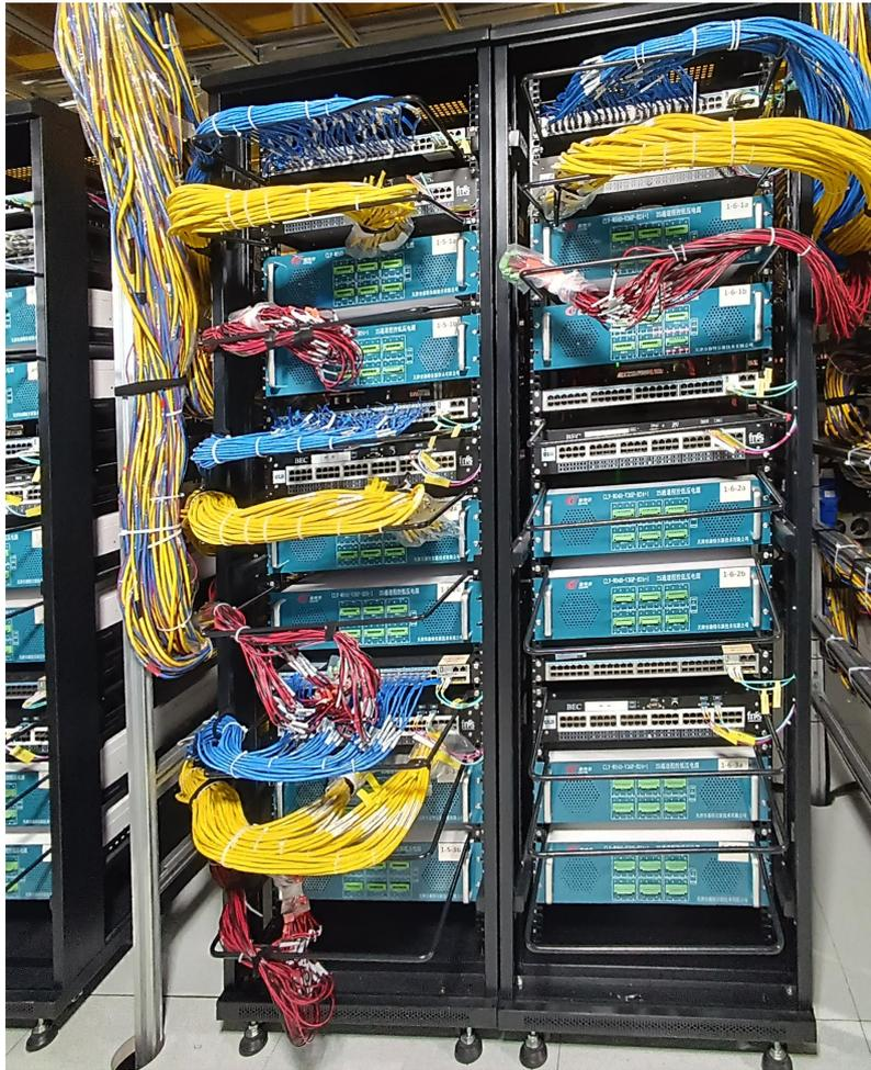
FIGURE 6.18: Three cables from UWBs to the lower power supply (Red/black pairs), the BEC (Yellow cable), and the DAQ switch (Blue cable).
